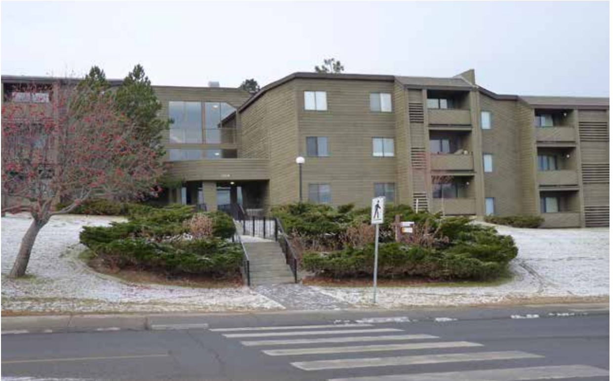
Condominium on Summit Drive - before.
